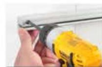
5. Loosen the set screws in the back 'D' that hold the glass display and place the completed display into the Rail 'B' and snug the set screws.
